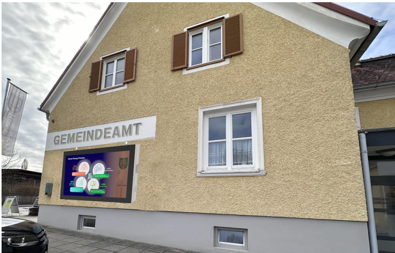
Figure 1 Exterior wall of the Gasen Municipality Building
